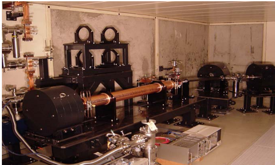
Figure 16. High-power setup for C-band accelerator structure testing at SPring8.
